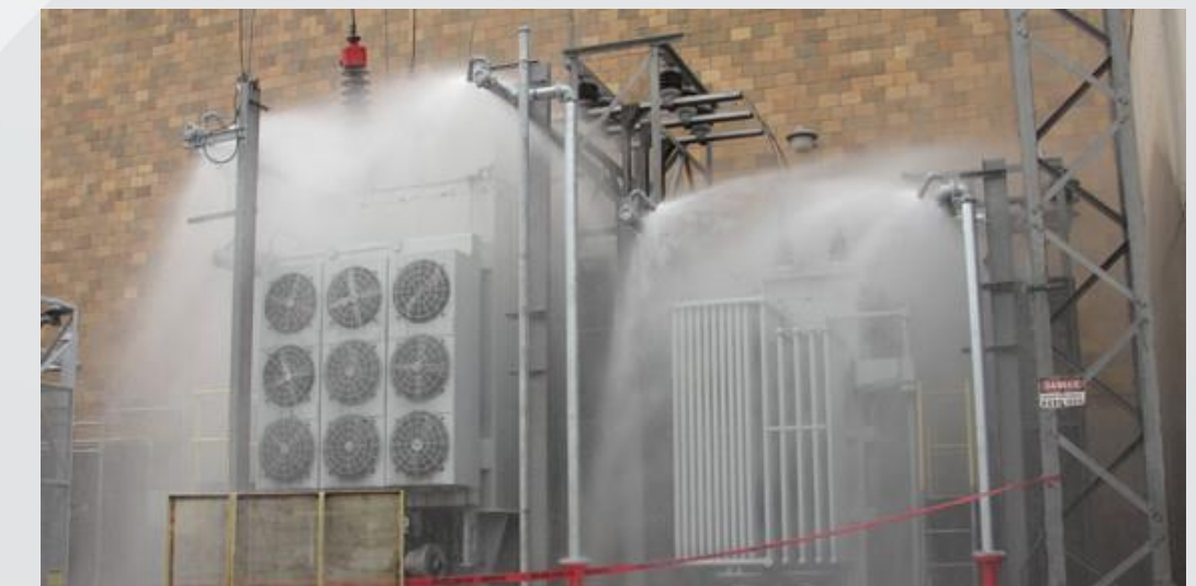
Water Spray System
