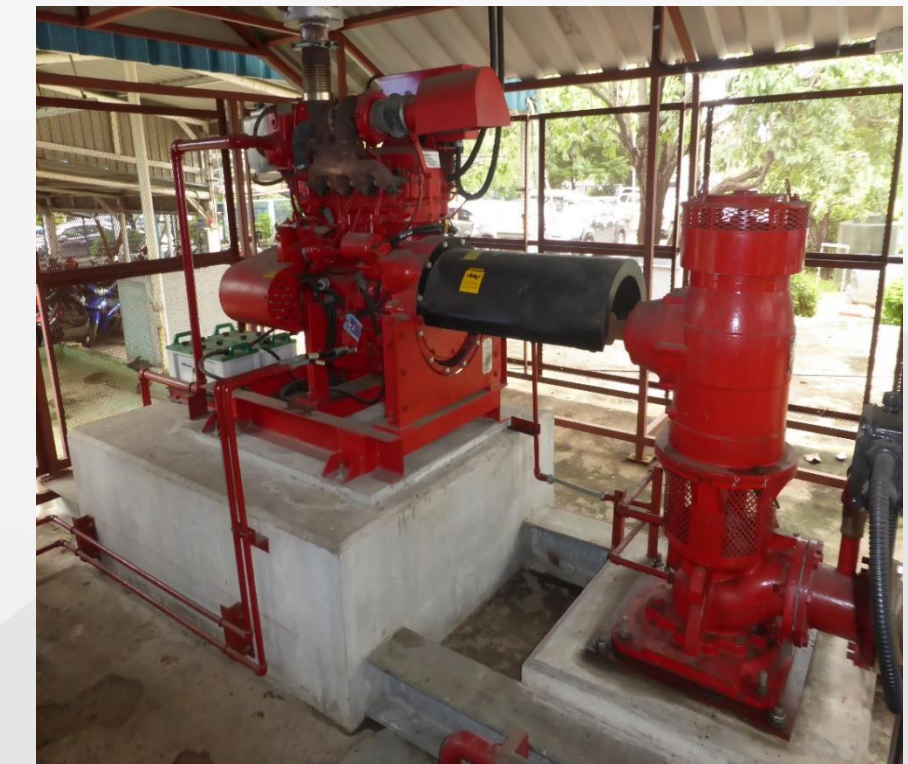
Vertical Turbine Fire Pump
