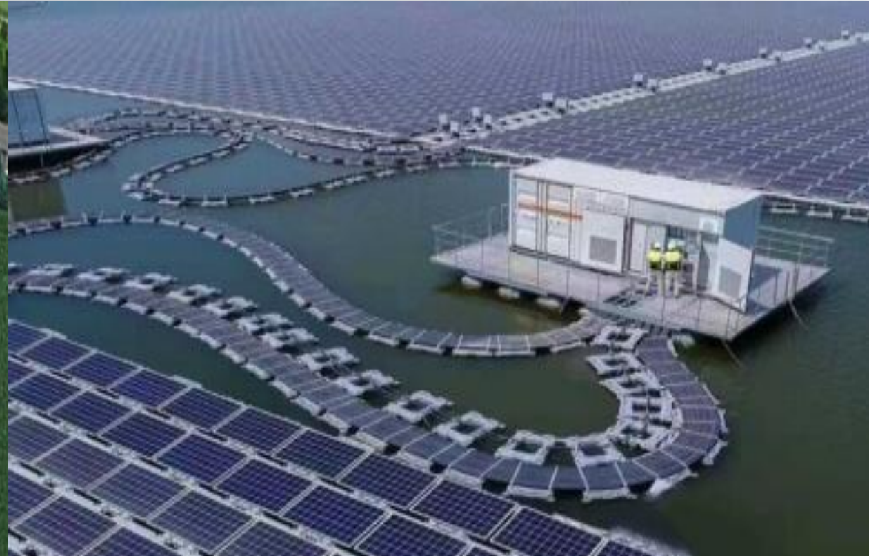
Floating Solar Farm
