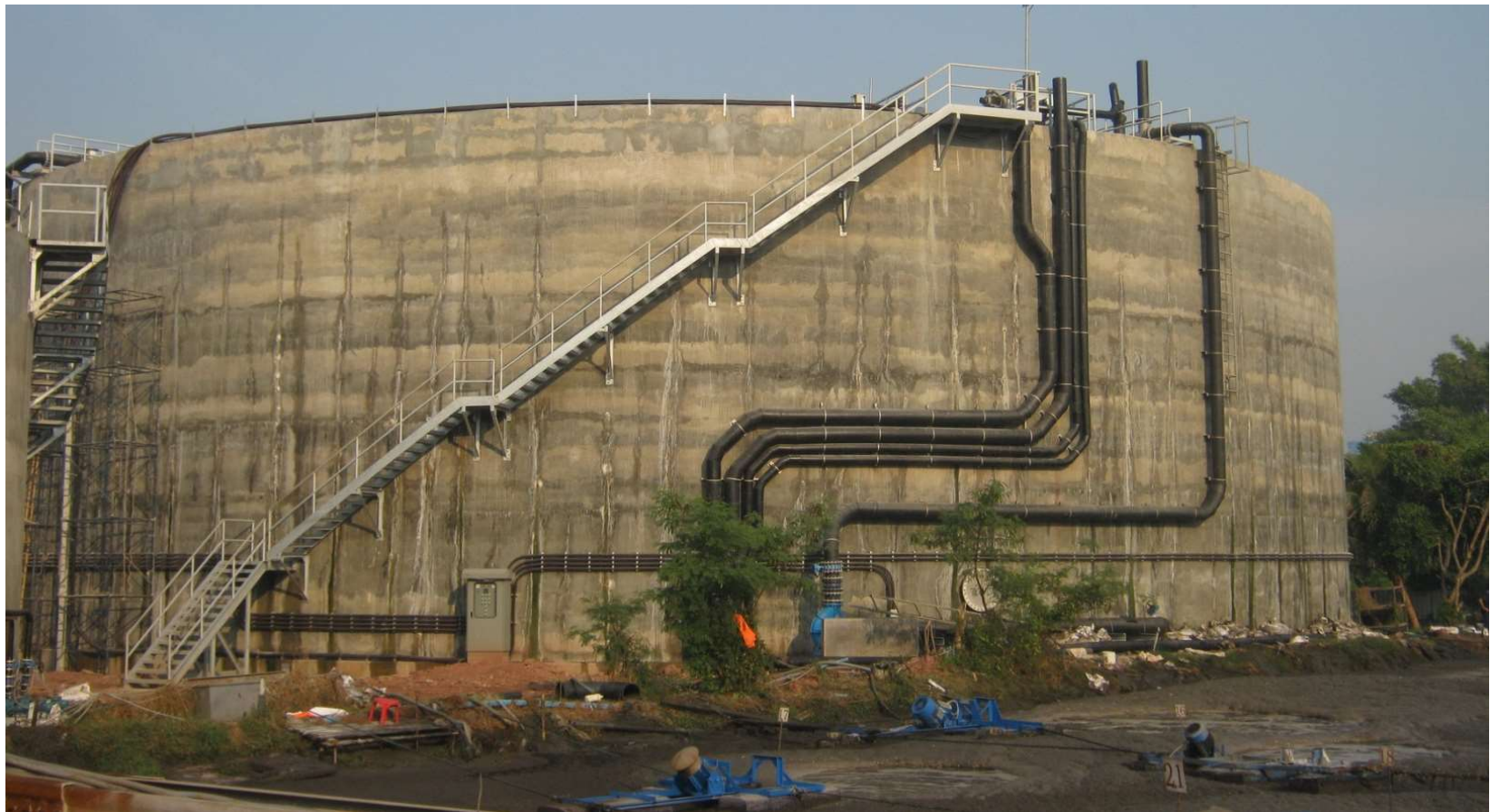
Crack on Waste-water Treatment Plant Wall
