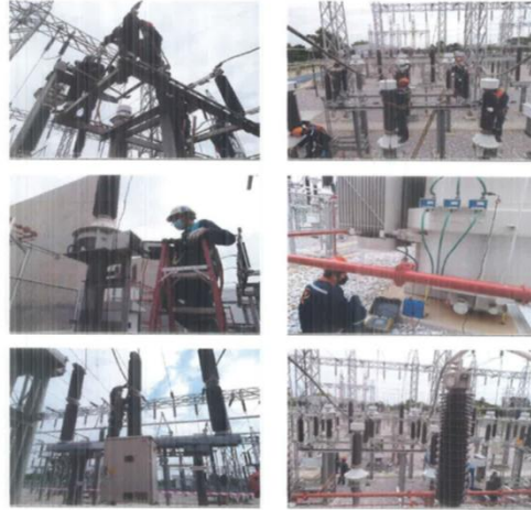
115 k V Switchyard are being inspected, tested and cleaned.
