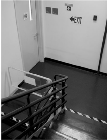
Interruption of exit stair at level of discharge. (Photo courtesy of Jake Pauls)
