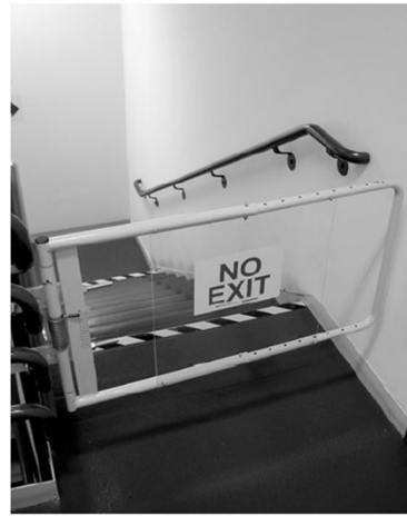
Sign on gate providing interruption of exit stair. (Photo courtesy of Jake Pauls)
