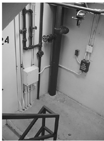
Fire protection and alarm equipment within, and penetrating the barrier walls of, an exit enclosure. (Photo courtesy of Jake Pauls)
