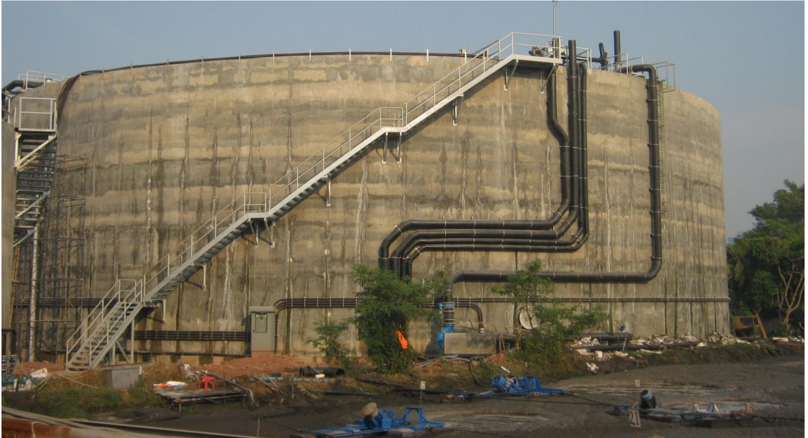
Crack on Waste-water Treatment Plant Wall
