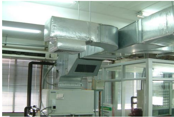
3.2 chilled-water air conditioning
