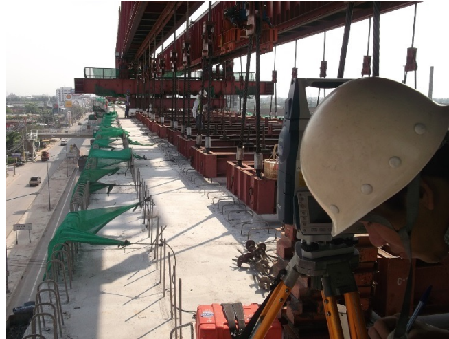
Span Alignment & Profile check
