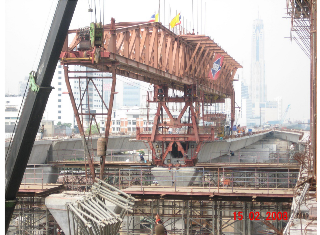
SVB Airport Rail Link by Overhead Gantry - STECON
