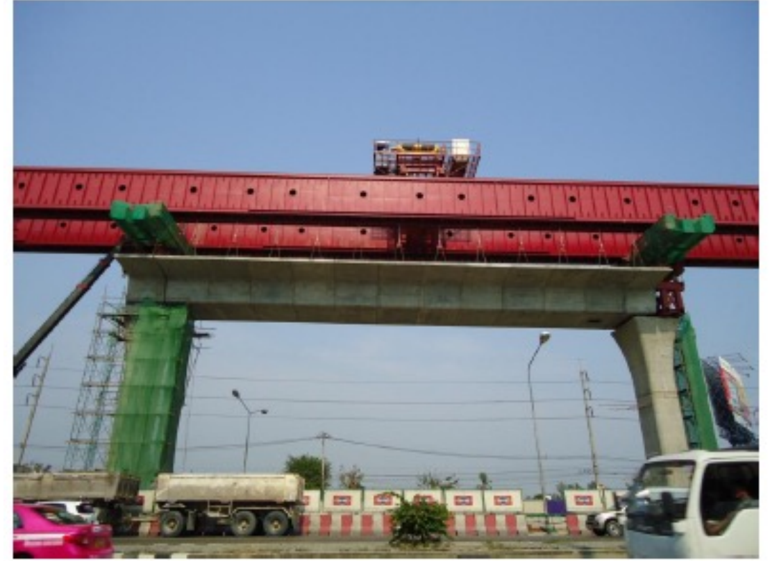
Figure A.6 Complete span assembly
