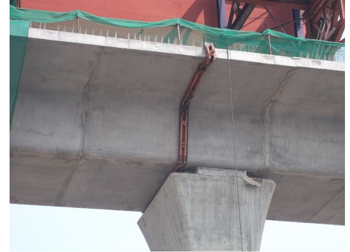
Concrete wet joint
