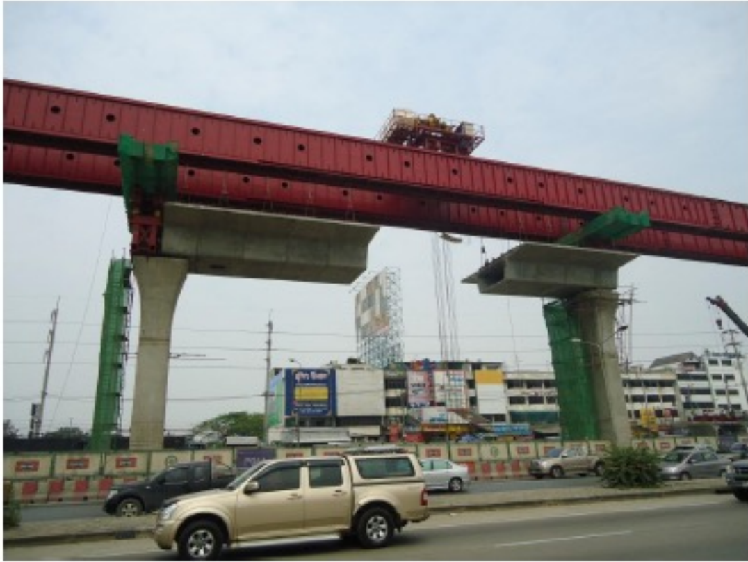
Figure A.5 Install segments 1, 2, 3, 10, 11, 12 then 4,5 (opposite side)
