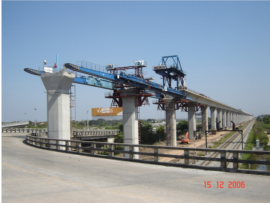
SVB Airport Rail Link by Underslung Gantry – STECON & VSL
