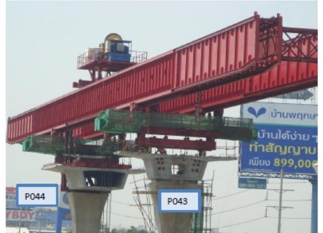
Figure A.2 Installing segment 1,2,3
