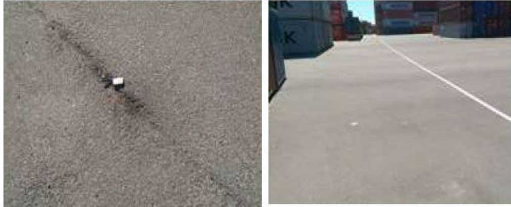
(a) Ravelling due to "open" texture (b) Dense uniform surface Figure 1-8 Un-controlled Deformation
