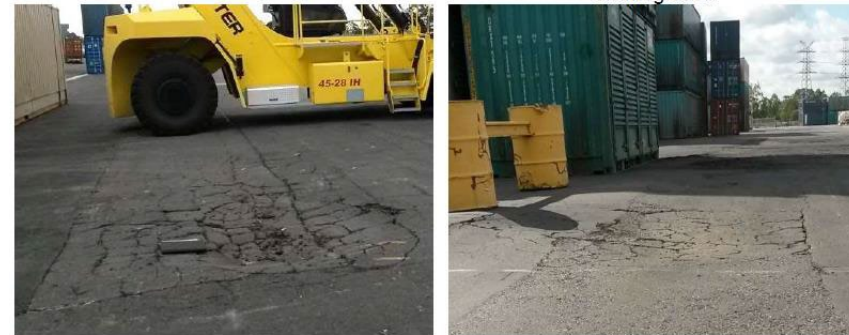
(c) Fatigue cracking with Surface Deformation (d) Fatigue cracking with Surface Deformation
