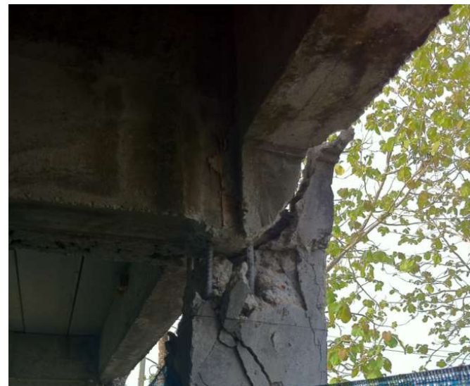
shear failure
