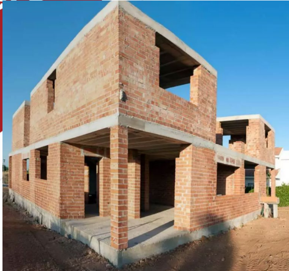
Wall Bearing system
