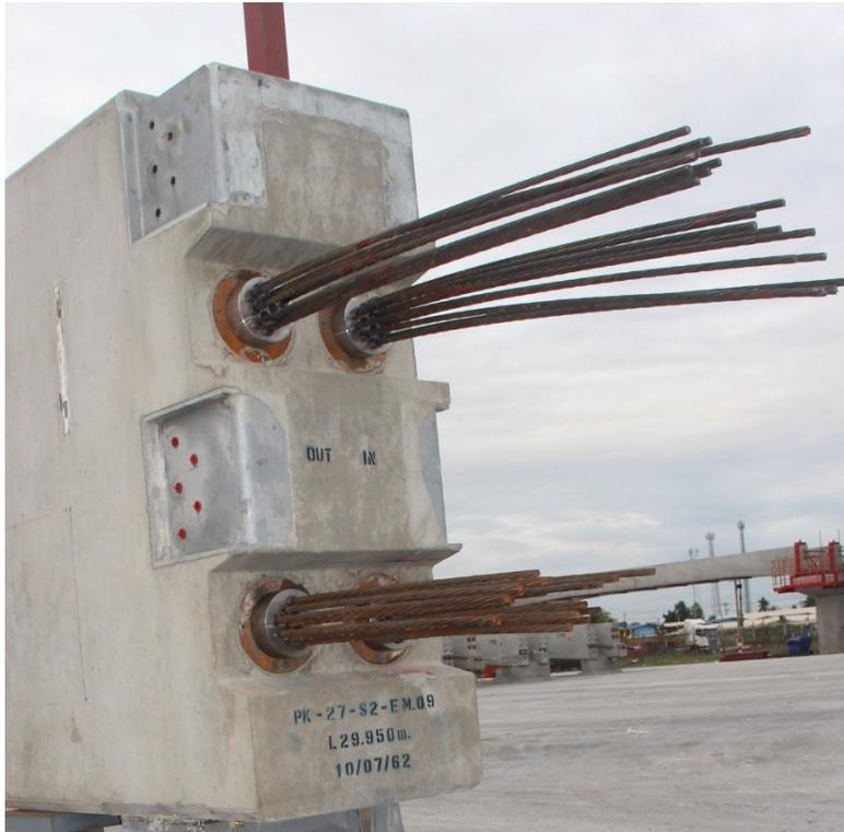
(7) Typical post-tensioning of the FPPC girder.
