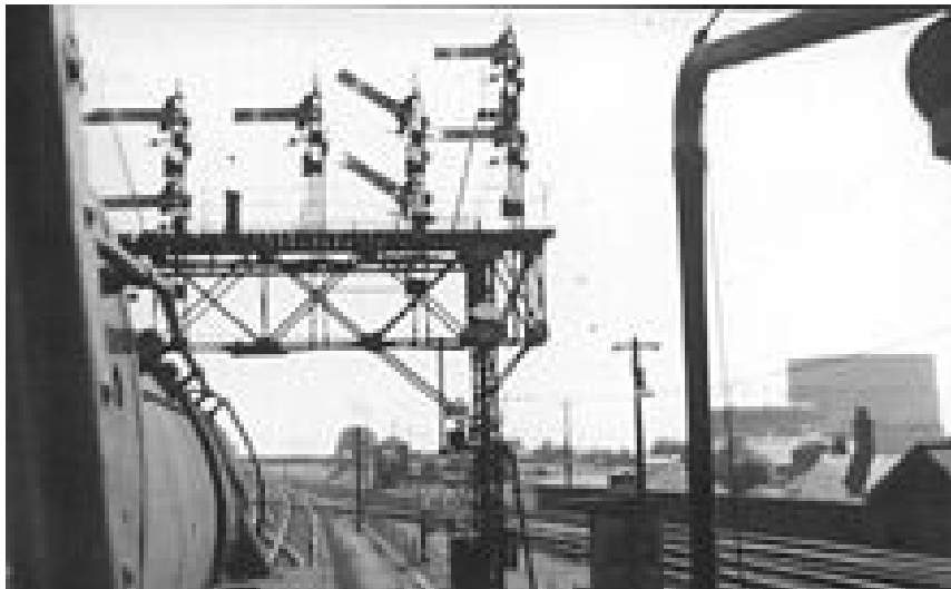
A gantry of British semaphore signals seen from the cab of a steam locomotive
