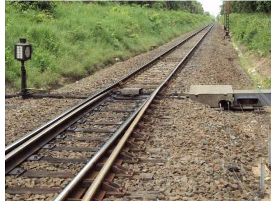
Mechanical Point Machine
