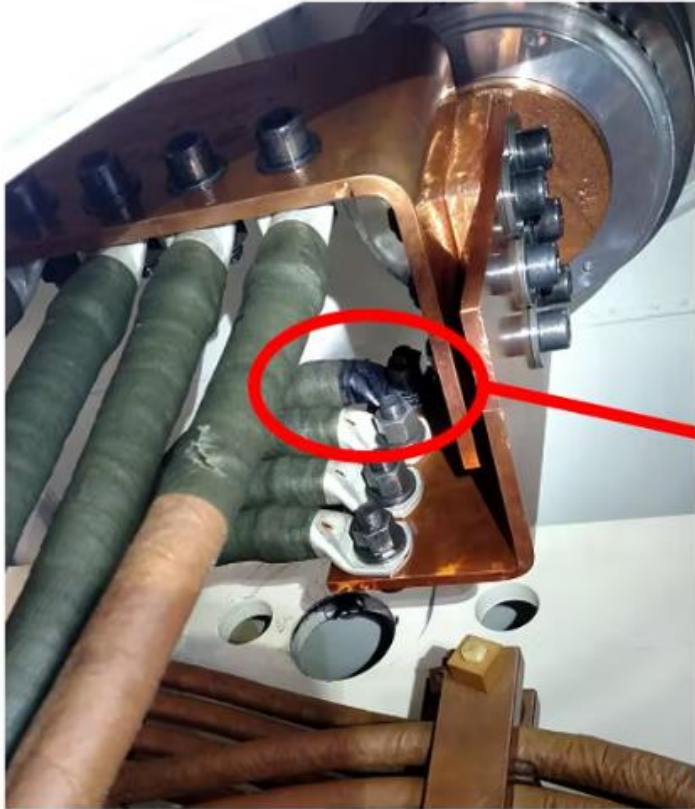
Figure 1. Hydrogen was generated in the transformer oil because of overheating on a low-voltage bushing connection owing to a loose nut on a 500-MVA generator step-up transformer. A hydrogen monitor alerted the owner to the problem. The transformer was repaired on-site.
