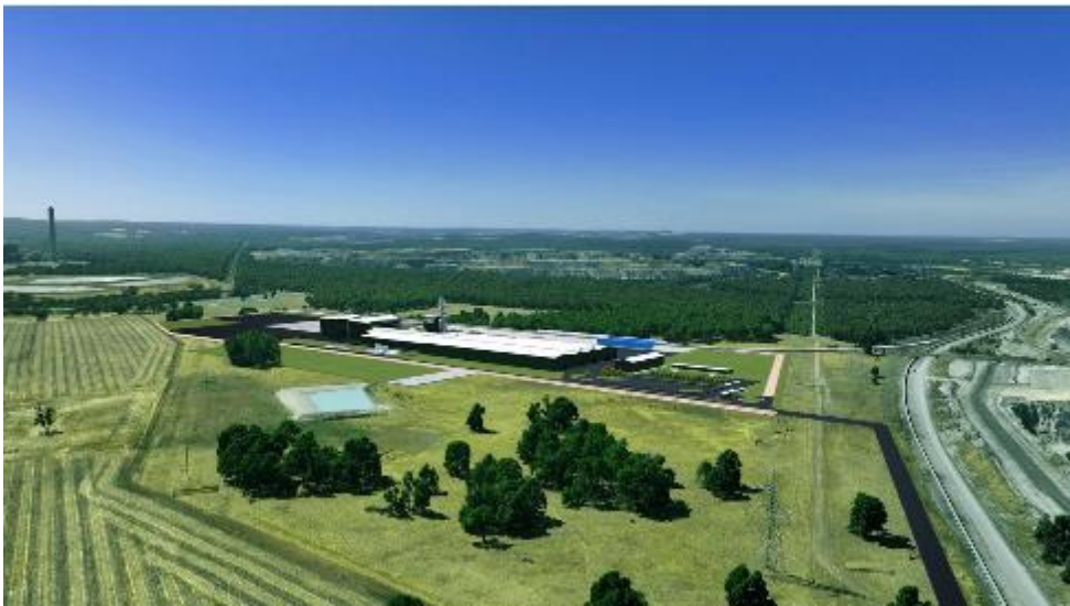
Green Steel of Western Australia's green steel recycling mill at Collie.
