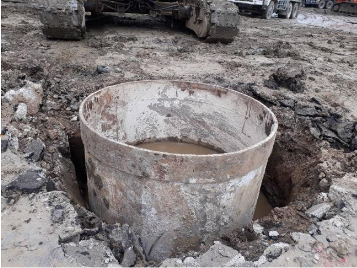
1. Outer casing installation
