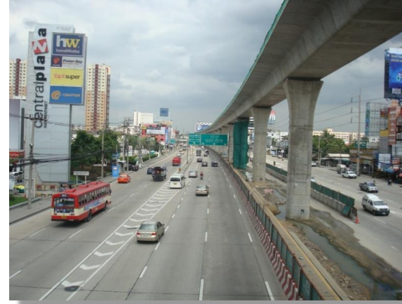
Barrettes supporting Purple Line MRT pier to reduce the size of the footing to be within the median
