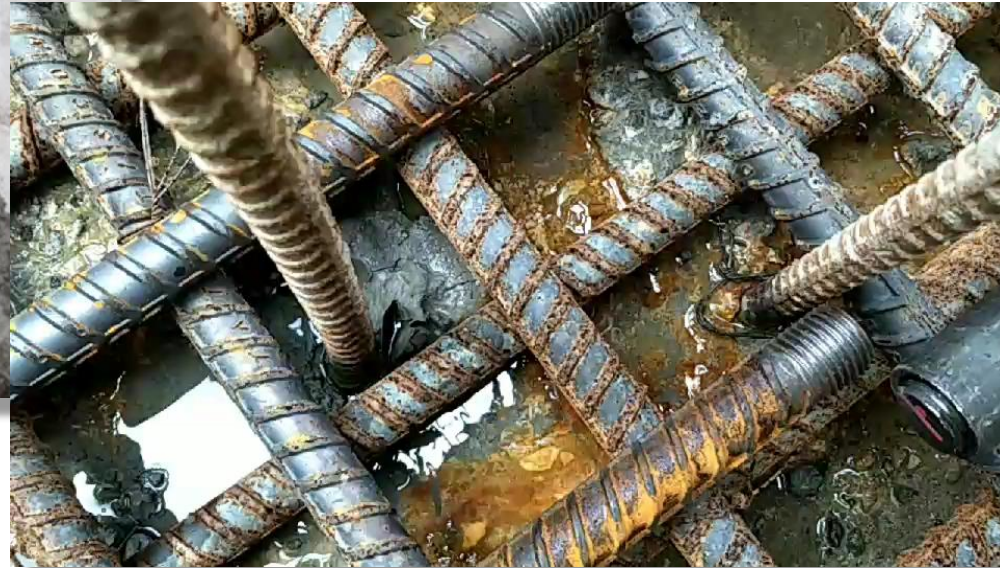
Channel water from pile head
