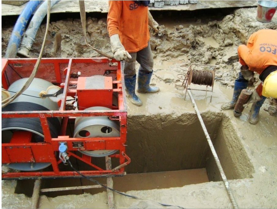
Drilling monitoring machine
