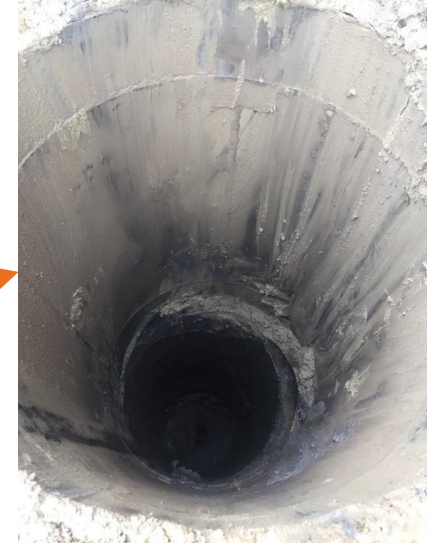
3. Inspection of pre-bored hole
