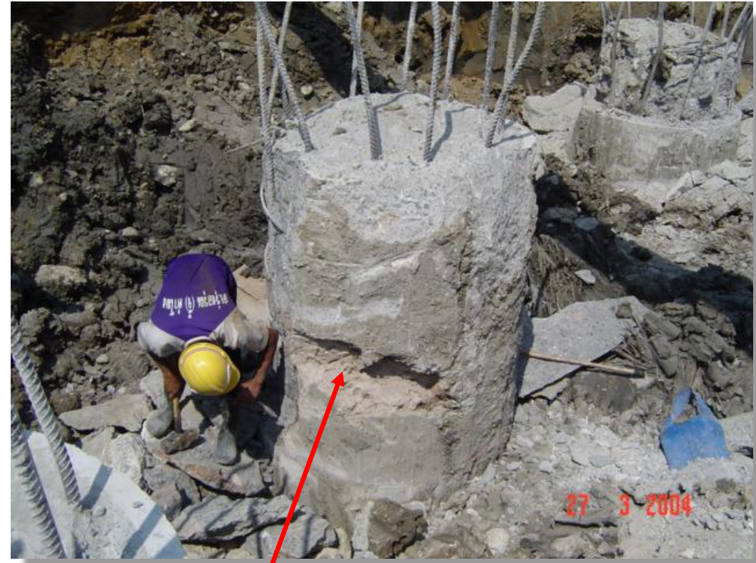
Contaminated concrete
