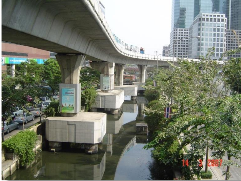
Bored piles supporting BTS pier with footing size likely to exceed the width of the road median
