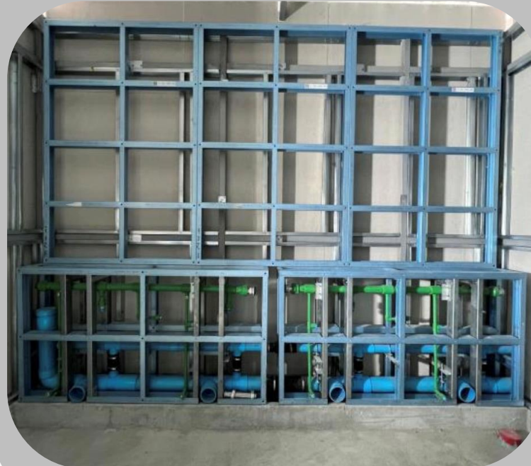
Installation (At site)
