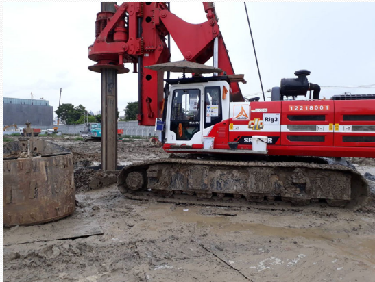
(2) Drilling by Auger
