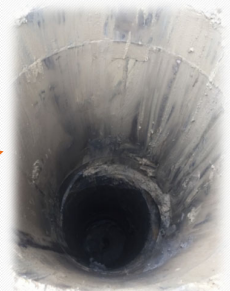
3. Inspection of pre-bored hole
