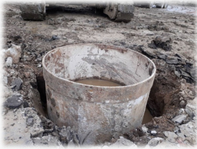
1. Outer casing installation
