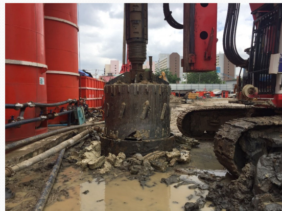
(3) Drilling by Bucket under slurry
