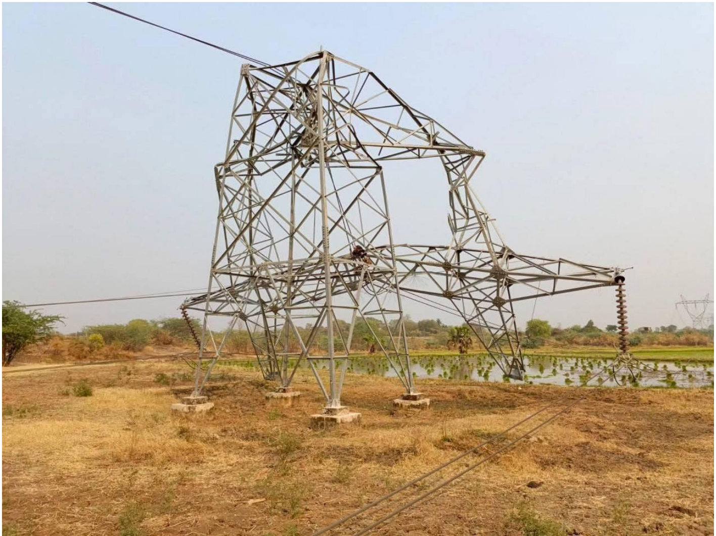
Failure of steel frame due to warping torsion
