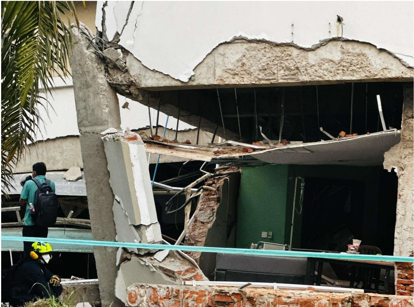
Failure of column due to captive effect
