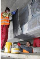
Shear strengthening
