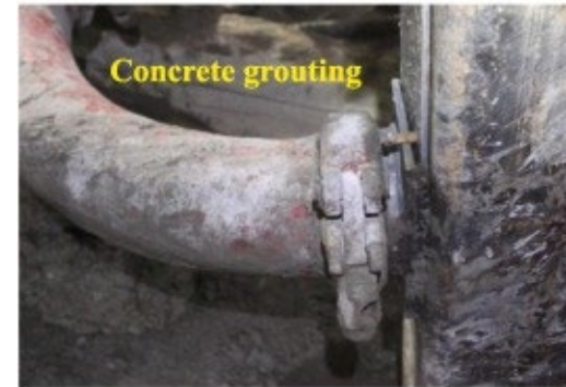
(c) CFST arch concrete grouting
