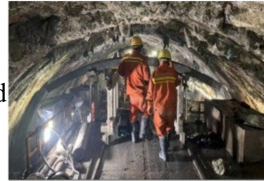
(a) TBM transportation platform
