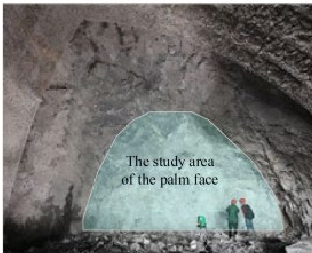
(a) Selection of research area for tunnel face analysis
