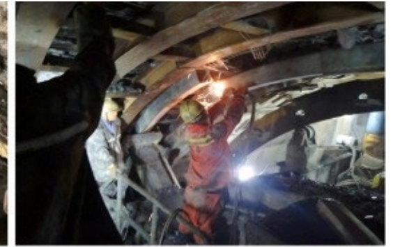
(b) CFST arch installation
