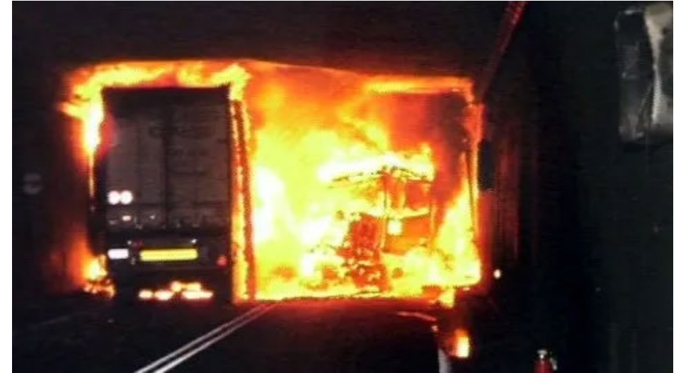
Fig: Swiss tunnel ablaze after head-on crash
