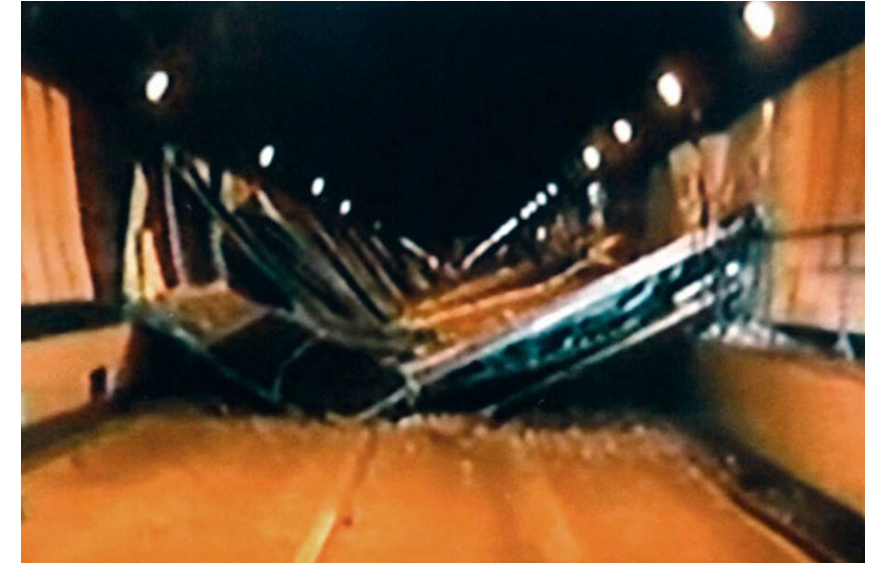
Fig: Broken concrete ceiling panels after collapsing inside Sasago Tunnel
