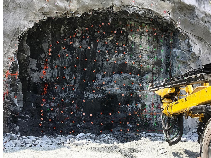
Figure 4 Sketch showing the drilling of blast holes after the completion of
