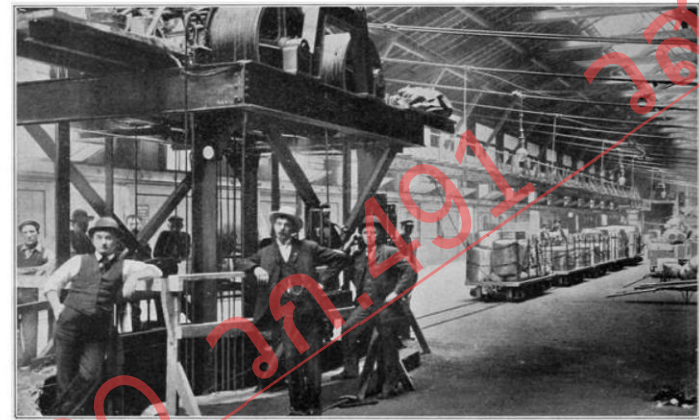
A specialized elevator from 1905 for lifting narrow gauge railroad cars between a railroad freight house and the Chicago Tunnel Company tracks below.
